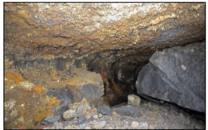
Fig. 2. Void 1 showing refluxed roof of a natural lava tube. The floor is the pipe roof.
