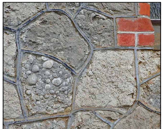
Fig. 3. The limestone blocks that were used for the church are of variable shape and size with many containing rich Pliocene mollusc fossil moulds and casts. The block on the left is dominated by trough shells (Mactridae) such as Eumarcia .
