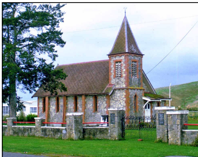
Fig. 2. St Luke's Anglican Church, Pakipaki, photographed in 1987, is made of local limestone, red brick facings and terracotta roof.
