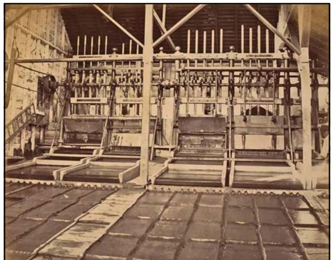
Fig. 4. The ore crushing stampers inside the Russell Battery.
