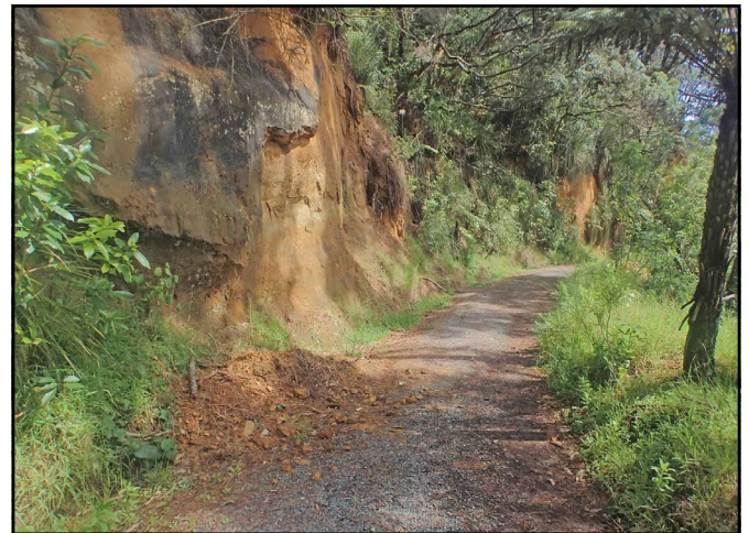
Fig. 2. That part of Edwin Mitchelson Track where the water table was blocked in 1965. Water poured over the outer edge in two places and was a major contributor to the tragic landslips.
