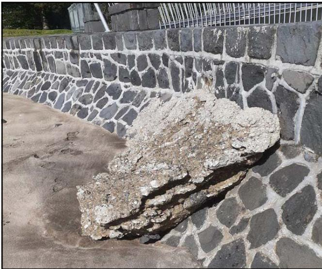
Fig. 3. Large “slug” of concrete against the basalt groyne, exposed when the sand was washed away from the west end of Mission Bay in 2020.
