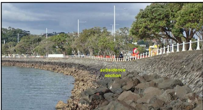
Fig. 2. View east along the outside of the Tamaki Drive causeway in the middle of Hobson Bay showing the subsided section above the buried Portland Rd–Newmarket stream valley. Photo: July 2020.
