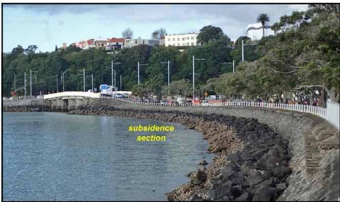
Fig. 1. View east along the outside of Tamaki Drive causeway showing the subsided section above the buried Purewa Stream valley, west of the bridge. Photo: July 2020.
