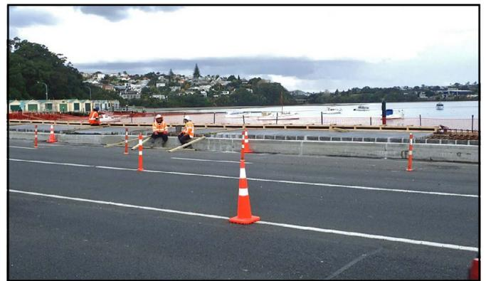
Fig. 3. Photo of work underway to raise the section of subsided Tamaki Drive where it crosses the buried Purewa Stream valley. Note the added 50 cm height of the new gutter. Photo: July 2020.
