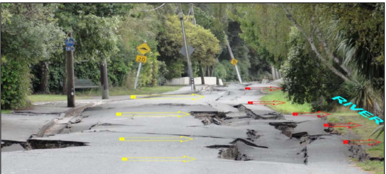
Lateral Spreading. (Cubrinovski et al. 2012)
