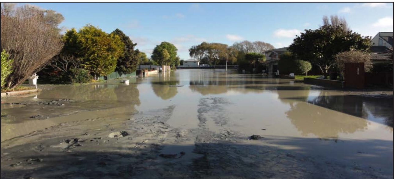
Liquefaction. (Photo: Brendon Bradley -UoC)
