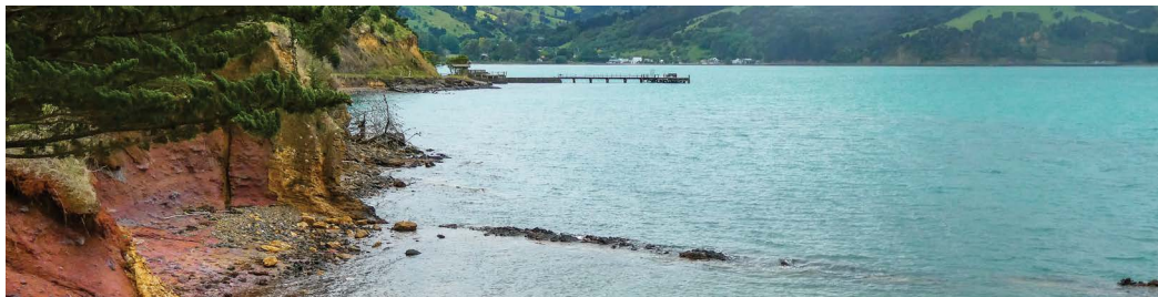
Looking north, a dyke and a wharf protrude into Akaroa Harbour on the Duvauchelle side. Photo credit: Janis Russell
