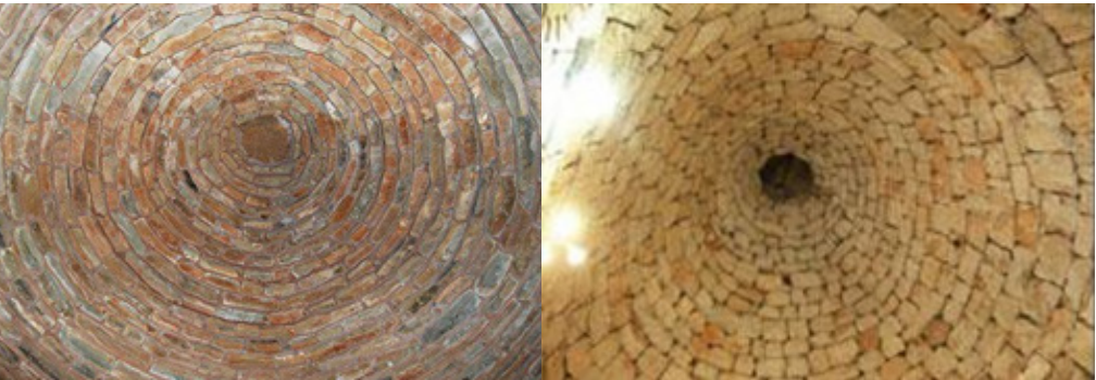
Corbelled houses inside view
