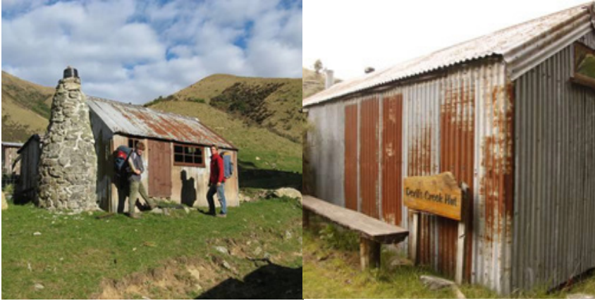
Old Corrugated Iron backcountry huts that many of us are familiar with. A mixture of stone and corrugated iron is used.
