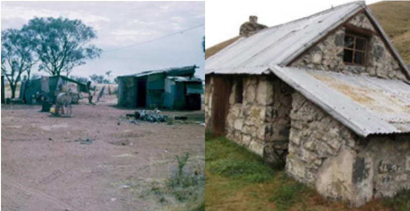
Corrugated iron dwellings, N.W. Queensland
