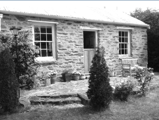
Renovated Stone cottage, Cromwell
