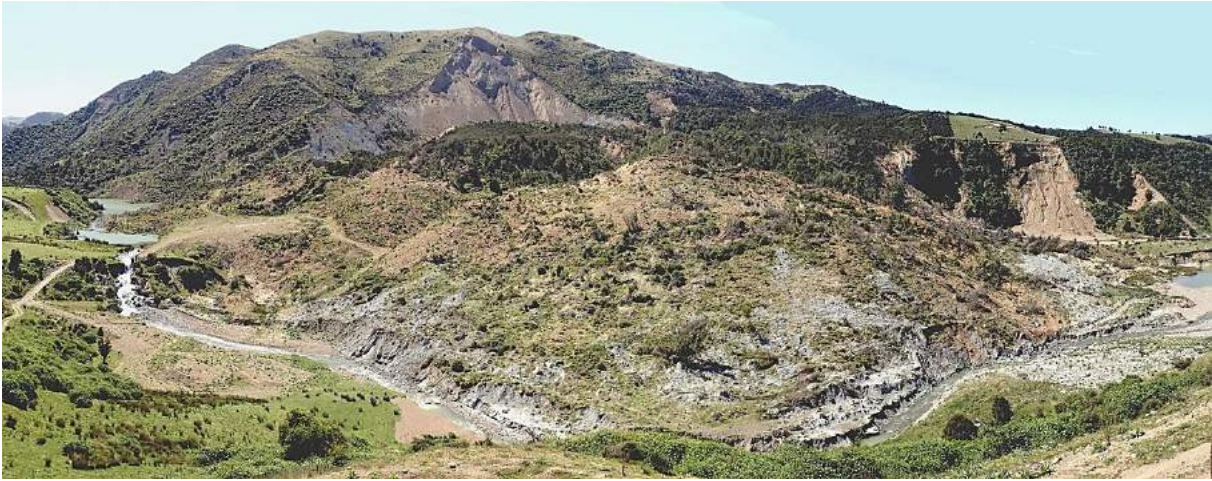
Fig. 5. A highlight of our Kaikoura Earthquake trip was the Leader River landslide and resulting dammed lake (far left).
