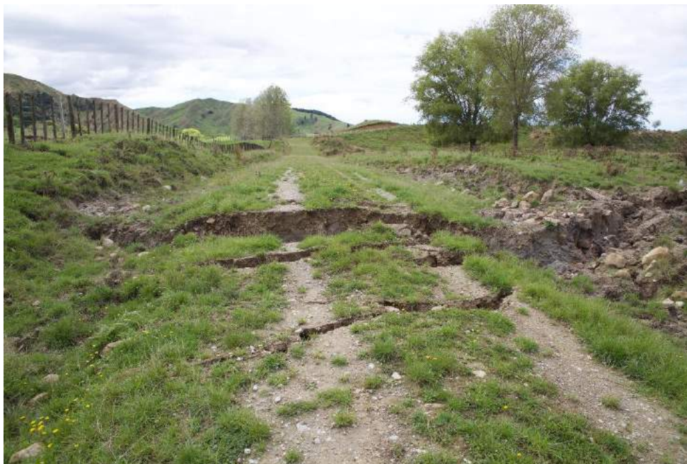
Figure One. Uplift and rupture on the boundary between the Uttings and Halls properties Waimata Valley 2016.
