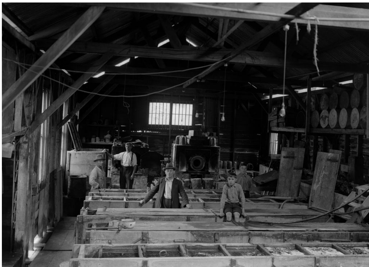
Figure 14. The zinc room, where the gold-cyanide liquid was piped through zinc boxes containing zinc filings. A thick slime rich in gold precipitated at the bottom of the boxes, and was collected regularly.
