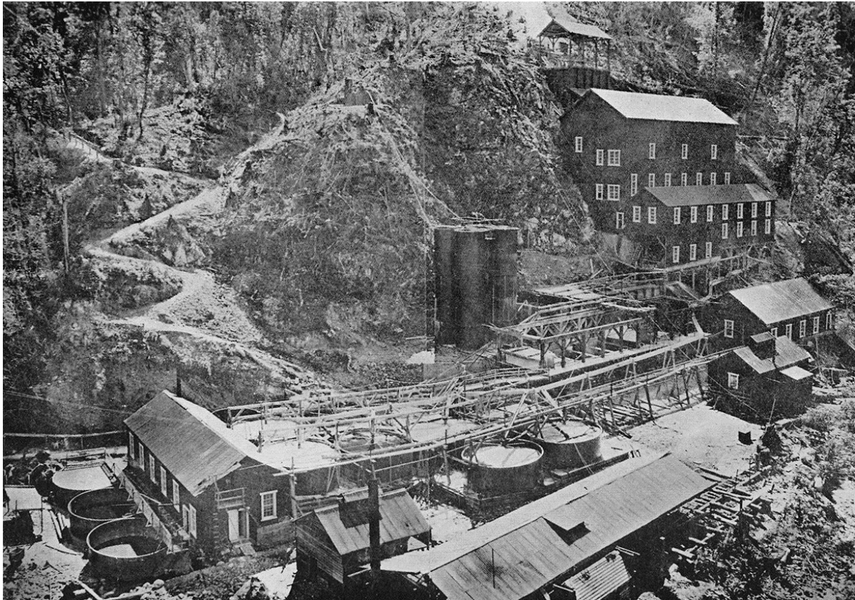
Figure 12: View across Snowy River, close to river level, showing the cyanide tanks and associated buildings in the foreground, taken about 1914. The cyanide tanks were later roofed over. Henderson (1917, p 172), Plate X
