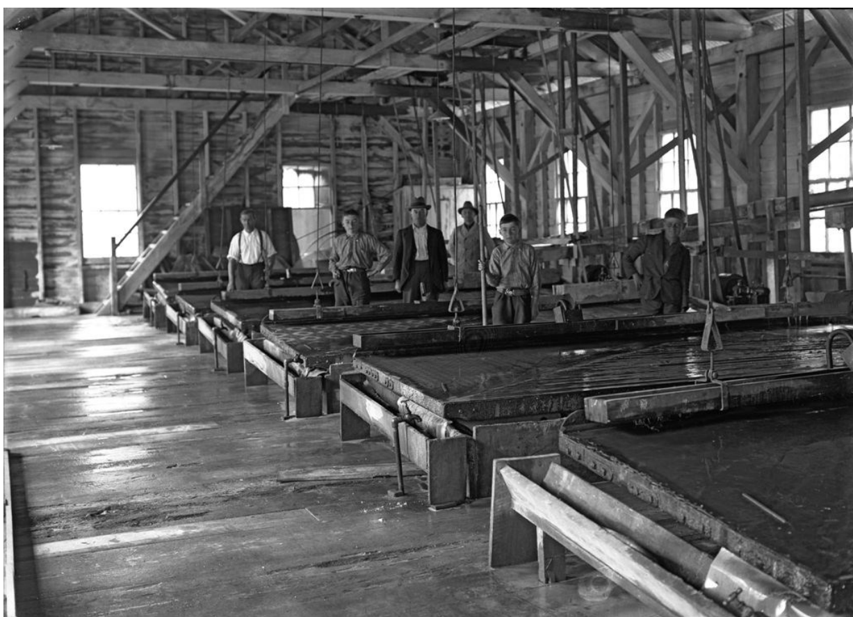
Figure 10. In the Wilfley room sands were washed across tables with riffles to concentrate heavier grains – largely gold and sulphides. The concentrates were again passed over amalgamating tables to catch any free gold, and then sent to the roasting furnace.
