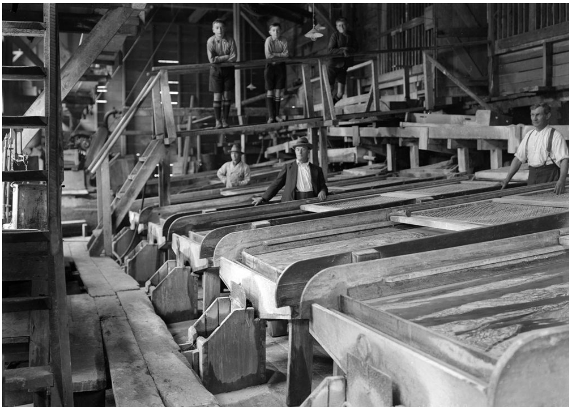
Figure 8. The plate room, where the slurry flowed over copper amalgamating plates coated with mercury. Fine gold amalgamated with the mercury, and was stuck to the coated plates. Alexander Turnbull Library, 1/2-233106-G
