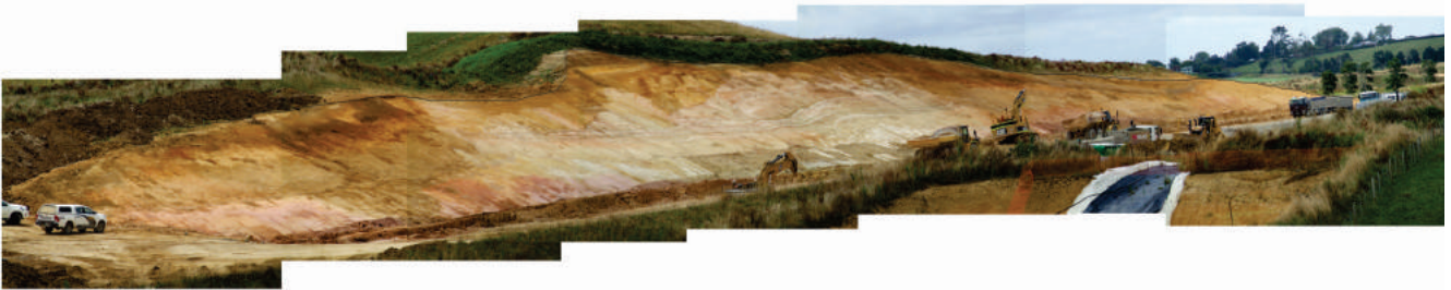
Figure 7: Osborne Road Expressway cutting site.
