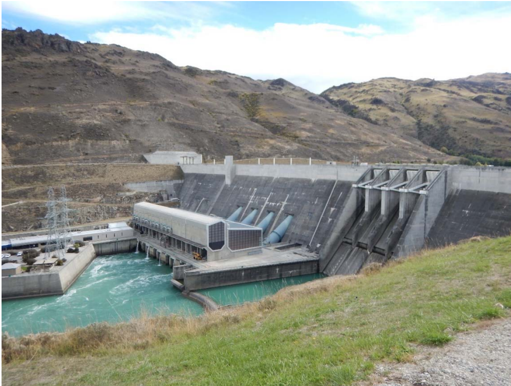
Figure 3: The Clyde Dam (Photograph by Mark Stirling)
