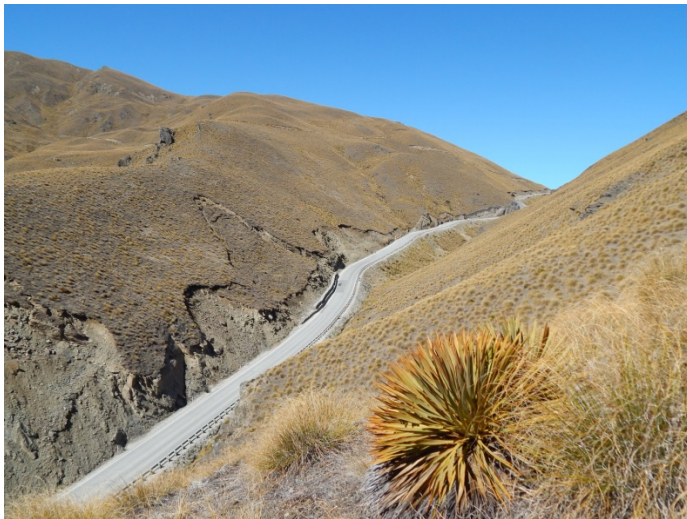
Fig. 15. Looking S from Chain Bay 3 towards the Crown Range Saddle
