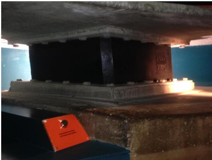
Figure 5. The rubber and lead ‘base isolators’ underneath Te Papa and many other buildings in Wellington. These act to ‘isolate’ the building from the ground to mitigate the shaking during an earthquake.
