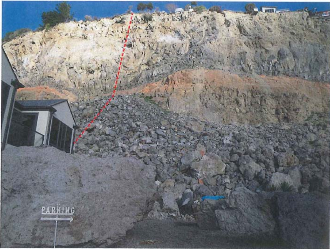
Figure 8 Photo showing runout adjacent to Section E
