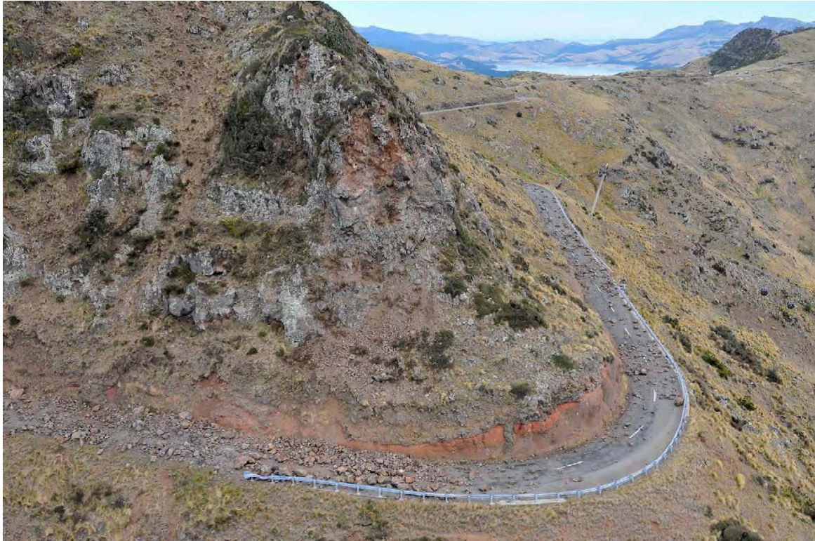
Figure 11 Rock fall analysis from controlled boulder release post September 2010 (from GNS Science). Rock falls on to Summit Road post 22 nd February 2011 (GNS Photo-GTH_5998, from GNS Landslide Reconnaissance Flight Immediate Report).
