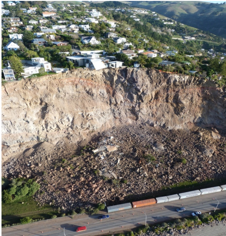
Figure 9 Cliff collapse at Clifton Hill following the 22 February and 13 June 2011 earthquakes - flown 14 June 2011. Note the partially collapsed house and use of ballasted shipping containers as temporary catch fences (Photo credit: Marlène Villeneuve/David Bell).
