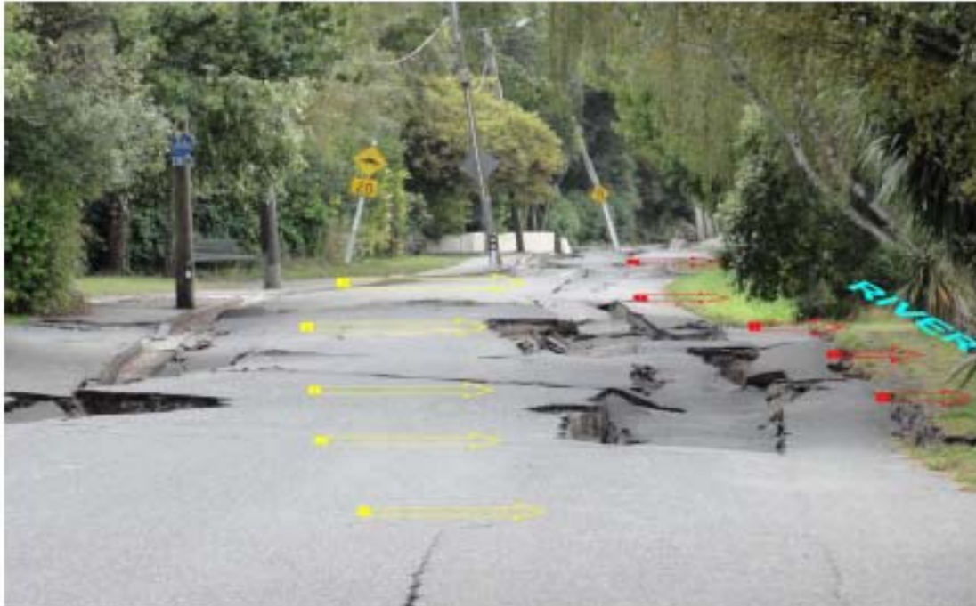
Figure 18 Lateral spreading toward the Avon Rivers (Fig 24 from Cubrinovski et al. 2011)
