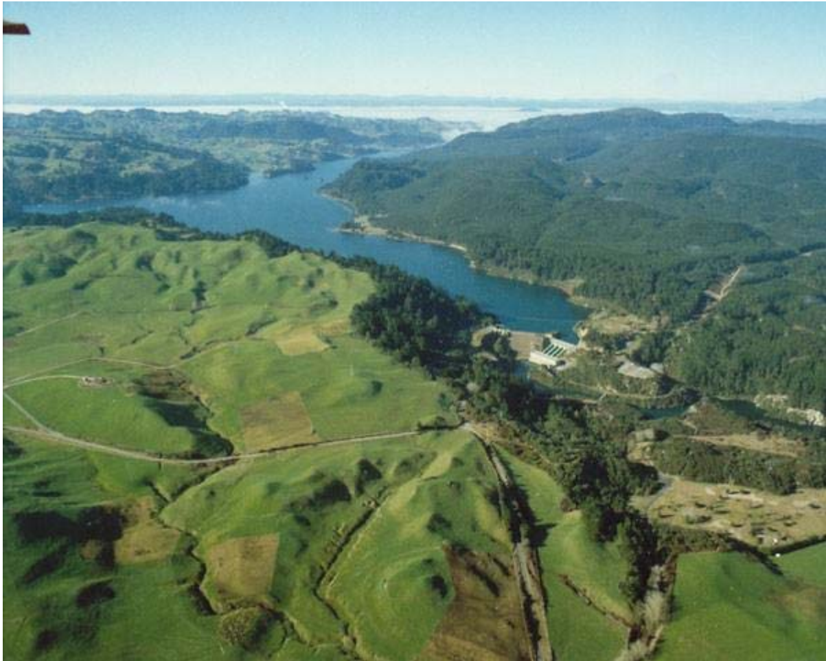
Figure 28: Ohakuri dam site on the Waikato River, forming Lake Ohakuri; with Maroa Volcanic Centre domes to the right and lumpy eroded partially hydrothermally altered Ohakuri Formation ignimbrite in the foreground. Photo L. Homer, GNS Science
