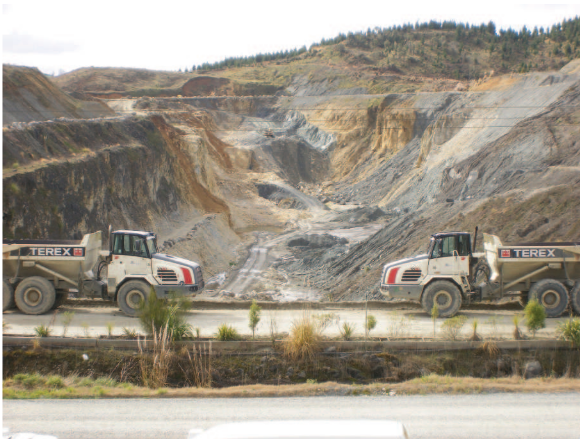
Fig. 15. Looking north into the Wairere Serpentinite Quarry along the trace of the Waipa Fault, with bounding Otorohanga Limestone (Lw) on left and Mahoenui/Mokau Group (Po/Pl) mudstone and sandstone on right.
