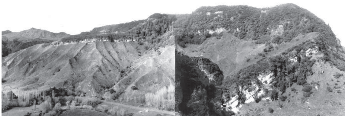
Fig. 18. Photo composite of the hill section on the southern side of the Awakino Tunnel, northern end of Awakino Gorge. Fig 19 shows the wider geological setting of this photo. From Kamp et al. 2004 (Fig. 11).
