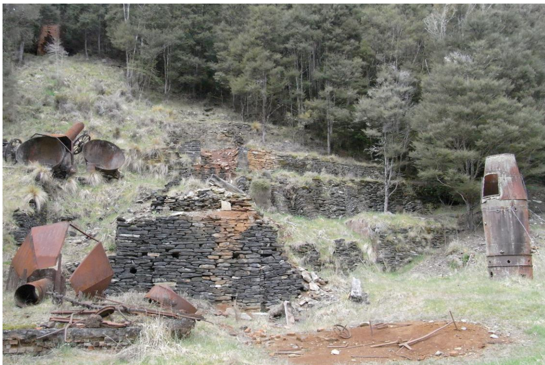
Figure 4.14 Smelter site in 2011. On the left are two roasting pots used to reduce the amount of sulphur in the ore before smelting. The hood of one of the roasting pots rests on the base of the smelter. The cylindrical structure on the right is the water jacket furnace used by the Champion Copper Company in 1886. Malita Limestone was used extensively to build both smelters. Photo: Mike Johnston
