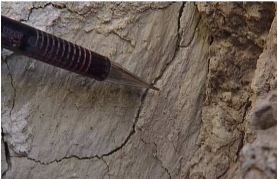
Figure 6: Detail of exposures in trench T00/3. Upper: Close-up of Fault 2, with at-fault vertical separation of at least 1.0 m. The fault displacement extends higher into the stratigraphic sequence than does Fault 1, and thus represents a separate, younger, rupture event. Lower: The pencil is perpendicular to steeply-pitching slickenside lineations on Fault 2. The lineations indicate oblique reverse-right lateral slip.
