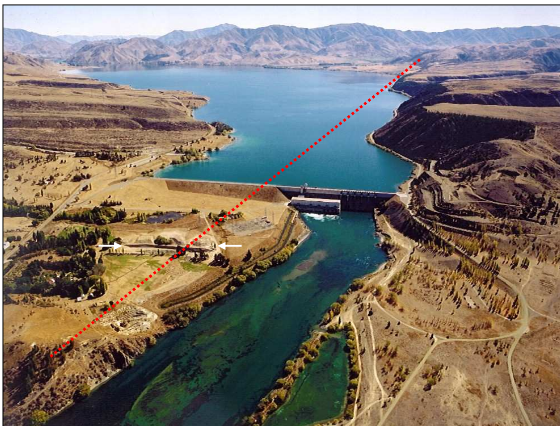
Figure 3: Aerial view NW across Aviemore Power Station. The powerhouse lies in front of the concrete gravity dam, with the grass-covered embankment dam to the left. Downstream of the dam are remnants of the ‘Aviemore’ alluvial terrace, with terraced alluvial fans to the far left. Note the approximate position of the Waitangi Fault (red line) and the large ‘Pinetrees’ (T01/1) fault investigation trench (white arrows). Photo: D.L. Homer, GNS Science.
