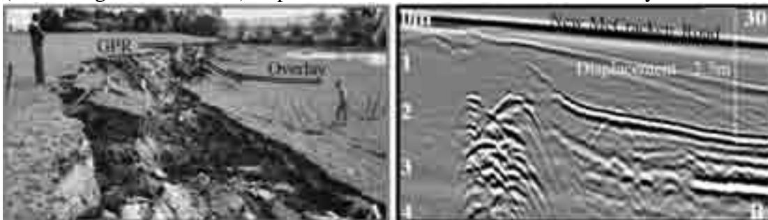
Figure 1: A) 1987 photo of Edgecumbe Fault 2.5m scarp north of McCracken Road. B) GPR detailing the rupture stratigraphy preserved under new McCracken Road.
