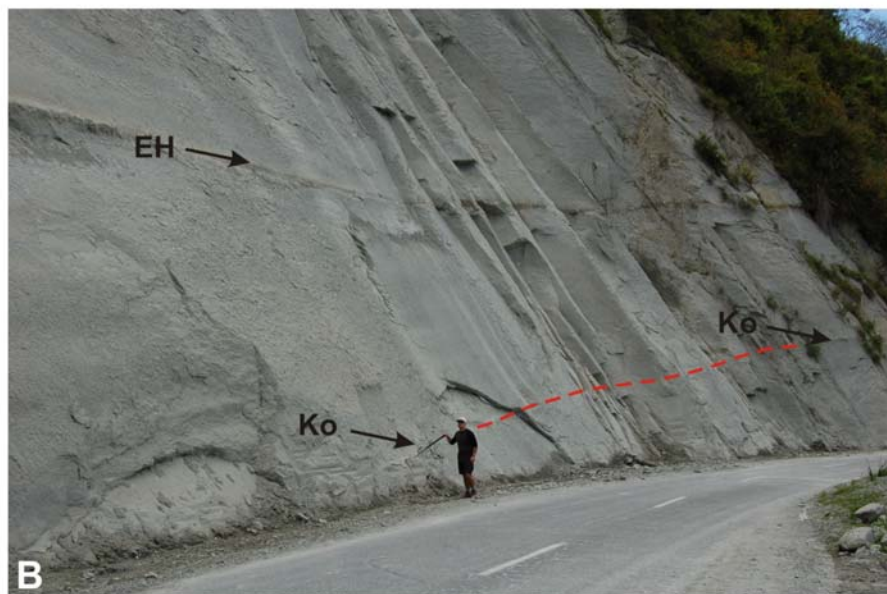
Figure 18. A. Eagle Hill Tephra (EH) and Kowhai (Ko) Tephra within Mangaweka Mudstone in the vicinity of Mangaweka township. A. As observed from the Rangitikei River Bridge; B. Cutting on south side of State Highway 54, 1.5 km east of Mangaweka township (Type Section, T22/517509, Naish et al. 1996). (Photos: B.V. Alloway ).
