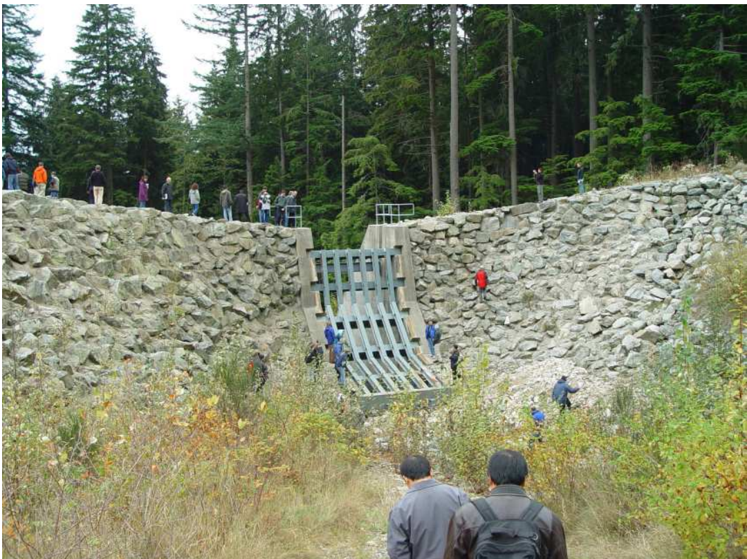
A debris-flow detention structure protecting a suburb of Vancouver, Canada, that may be a suitable model to trap debris-flow boulders in the former quarry area of Awatarariki Stream.
