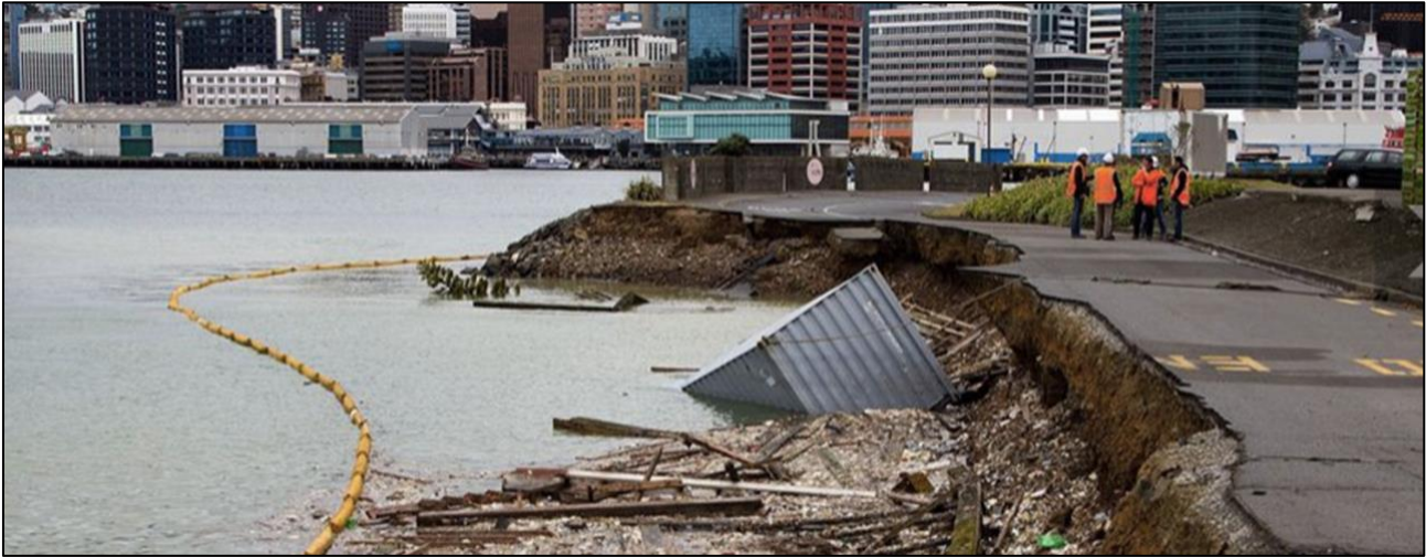
Damage to port facilities in Wellington during the 2016 Kaikōura earthquake. Understanding how quickly infrastructure can recover from similar events, and the implications for further earthquakes during the recovery is critical to inform disaster risk planning for earthquake sequences.
